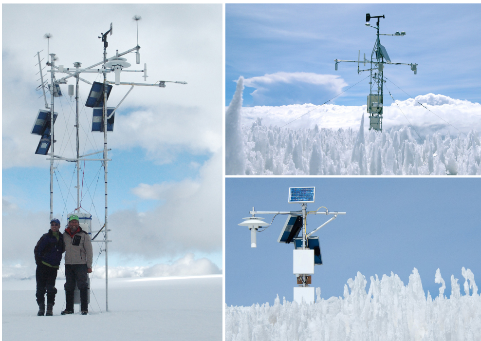
Figure 1. AWS on Quelccaya (left) and Kilimanjaro (right; stations are adjacent to one another). The Quelccaya tower and one of those on Kilimanjaro are custom, modular designs of aluminum tubing and structural fittings. Recently, radiation shields compatible with the U.S. Climate Reference Network (USCRN) began operating at both sites, visible in images as large white disks with vertical tubes beneath; these house 3 PRTs each to measure temperature and a Vaisala HMT337 for humidity measurement.
