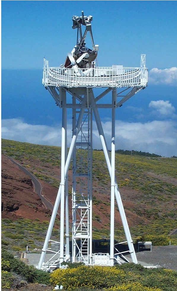
Figure 1: Dutch Open Telescope (DOT) with full fold-down 7 m diameter dome enclosure. Left: enclosure fully open, leaving the telescope in a desired natural wind flow. Right: enclosure closed in winter - note the substantial snow and ice build-up on the ladder and elevator frame work, but not on the dome – it slides off naturally.
