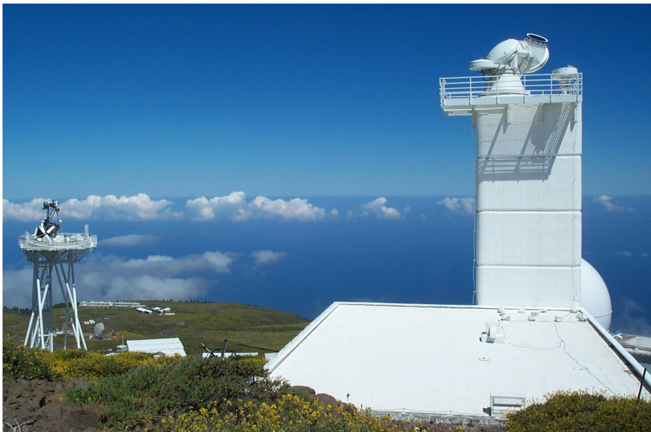
Fig. 1. The Swedish Solar Telescope (SST) at the Observatorio del Roque de los Muchachos (ORM) at an altitude of 2360 m. The area is free to the ocean between west (left) and north-east. Wind speeds of just a few m/sec (e.g. 2 m/sec) up till 20 m/sec from over the ocean or from over a layer of clouds above the ocean permit excellent seeing conditions. The relatively slender tower of 17 m height (right) has on top the so-called Turret, which consists of an entrance lens of 108 cm – clear aperture 97 cm – and two folding mirrors under 45° of 1.4 m diameter. This system directs the light downward through a steel tube in the tower to an optical lab in the basement of the building. The light path from the entrance lens to the optical lab is evacuated to eliminate image disturbance from air-temperature fluctuations inside the telescope. The entrance window is visible as a black ellipse on top. The Turret is made as compact as possible around the optical beam. Consequently, its outside shape shows the two folding mirrors under 45° with one pivot-joint with the horizontal axis – the elevation axis – between the two mirrors and another pivot-joint with the vertical axis – the azimuth axis – just underneath the second mirror. The flat round piece to the left is a counterweight to balance the azimuth axis. The lid to cover the entrance lens can be seen with its support system on top of the tower at the very right. At the left side of the picture one can just see the Dutch Open Telescope (DOT), likewise a high-resolution solar telescope, but with a contrasting principle: the primary light beam 'inside' the telescope is as open as possible for air flushing by natural wind. Both principles prove to be very successful on La Palma. Despite the telescopes' difference in principle, the SST gears are a further development of these of the DOT.
