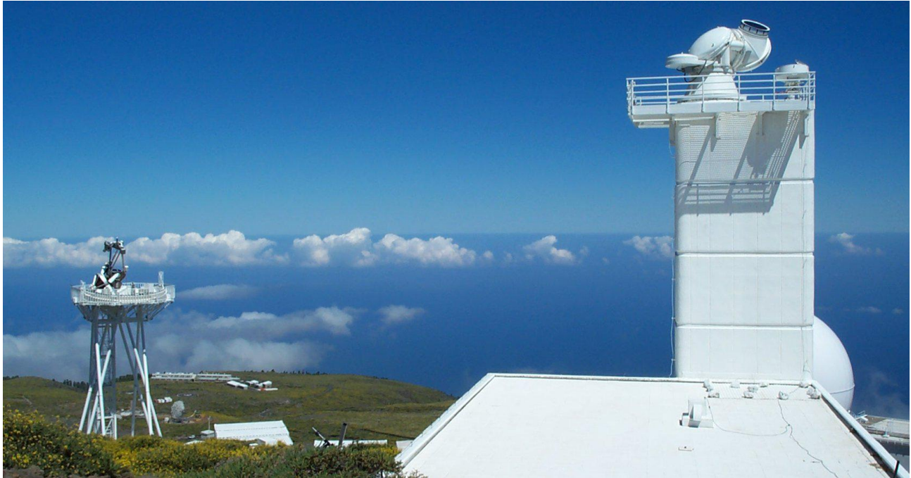
Fig. 5. The Swedish Solar Telescope (SST) at the Observatorio del Roque de los Muchachos (ORM) at an altitude of 2360 m. The area is free to the ocean between west (left) and northeast. Wind speeds of just a few m/s (e.g. 2 m/s) up till 20 m/s from over the ocean or from over a layer of clouds above the ocean permit excellent seeing conditions. The relatively slender tower of 17 m height (right) has on top the so-called turret, which consists of an entrance lens of 108 cm – clear aperture 97 cm – and two folding mirrors under 45^\circ of 1.4 m diameter. This system directs the light downward through a steel tube in the tower to an optical lab in the basement of the building. The light path from the entrance lens to the optical lab is evacuated to eliminate image disturbance from air-temperature fluctuations inside the telescope. The entrance window is visible as a black ellipse on top. The turret is made as compact as possible around the optical beam. At the left side of the picture one can see the Dutch Open Telescope (DOT), likewise a high-resolution solar telescope, but with a contrasting principle: the primary light beam 'inside' the telescope is as open as possible for air flushing by natural wind. Both principles prove to be very successful on La Palma.
