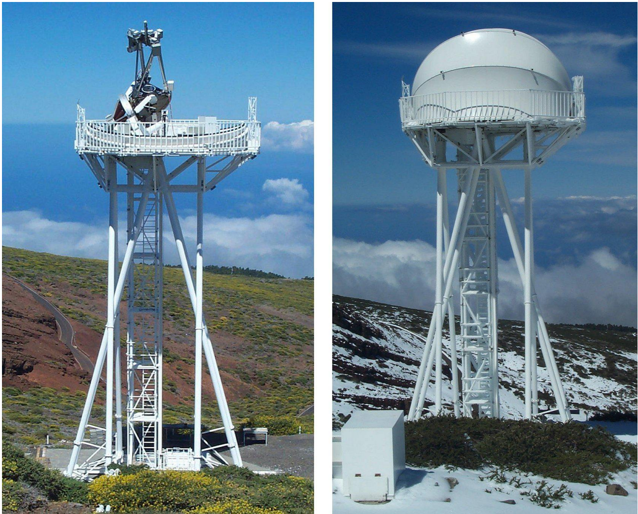
Fig. 2. Dutch Open Telescope (DOT) on La Palma. Left : tent dome open for solar observations. Right : tent dome closed during wintertime with ice in ladder/elevator framework. Practically no ice sticks on the tent cloth due to its smooth coating. The viewing direction in this photograph corresponds with the scheme of fig. 1b.
