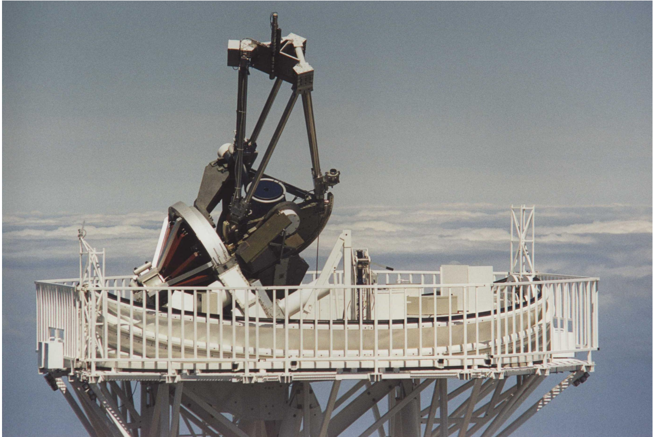
Fig. 6. Close-up of the DOT on the tower platform. The primary mirror and the optical beam to the primary focus are fully open to wind. The DOT was the first telescope showing that such an open-air path can permit diffraction-limited resolution. Note that the primary mirror is located well above the declination axis of the equatorial mount. It sticks out high above the platform into full wind flushing.
