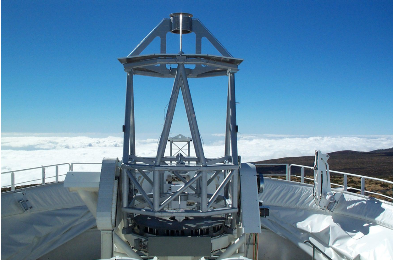
Fig. 6. The GREGOR telescope structure with open dome seen from the inside.
