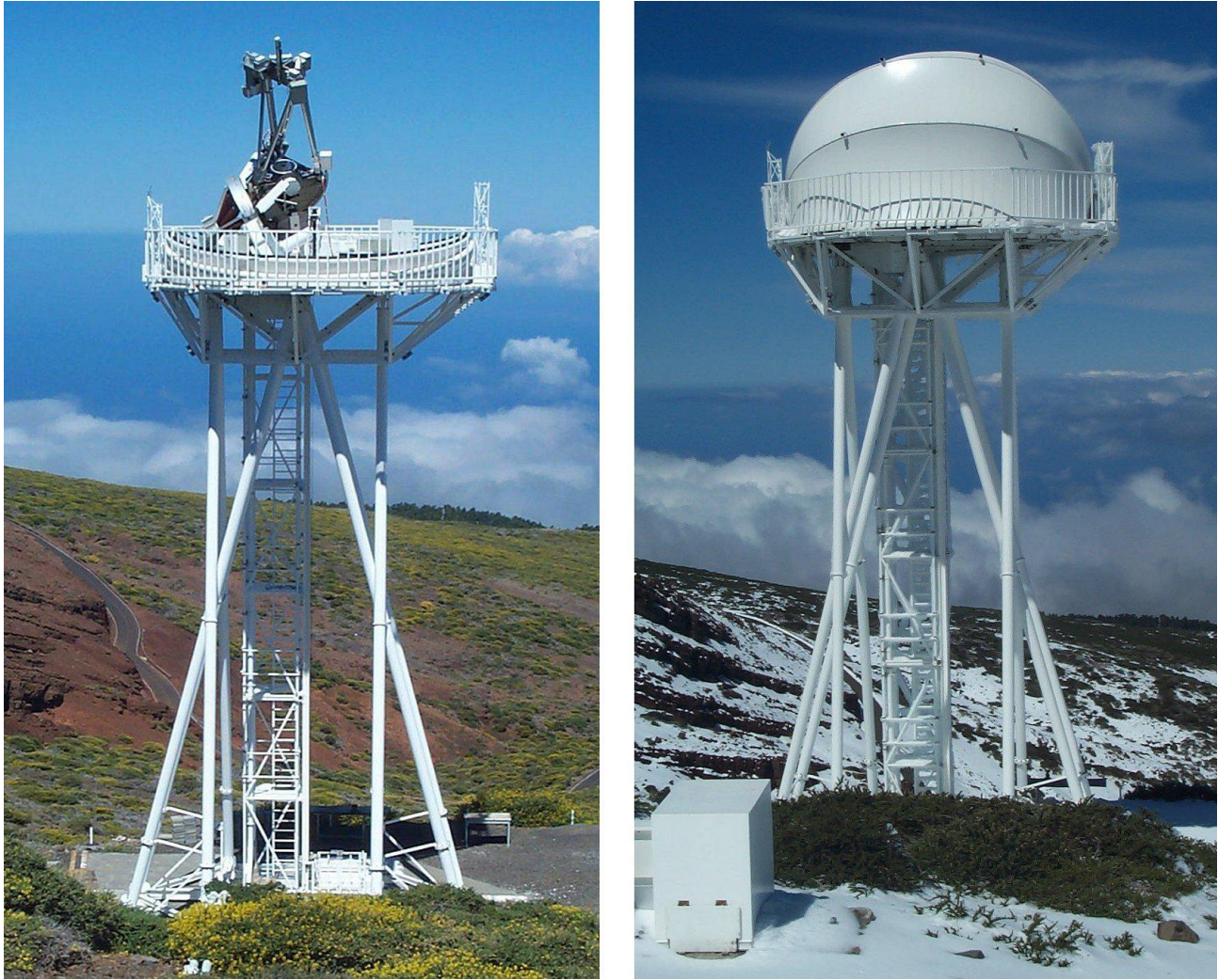
Fig. 2. The Dutch Open Telescope (DOT) on La Palma. Left : open dome for solar observations. Right : closed dome in winter; there is ice in ladder/elevator framework, however practically no ice sticks on the cloth due to its smooth outside coating.
