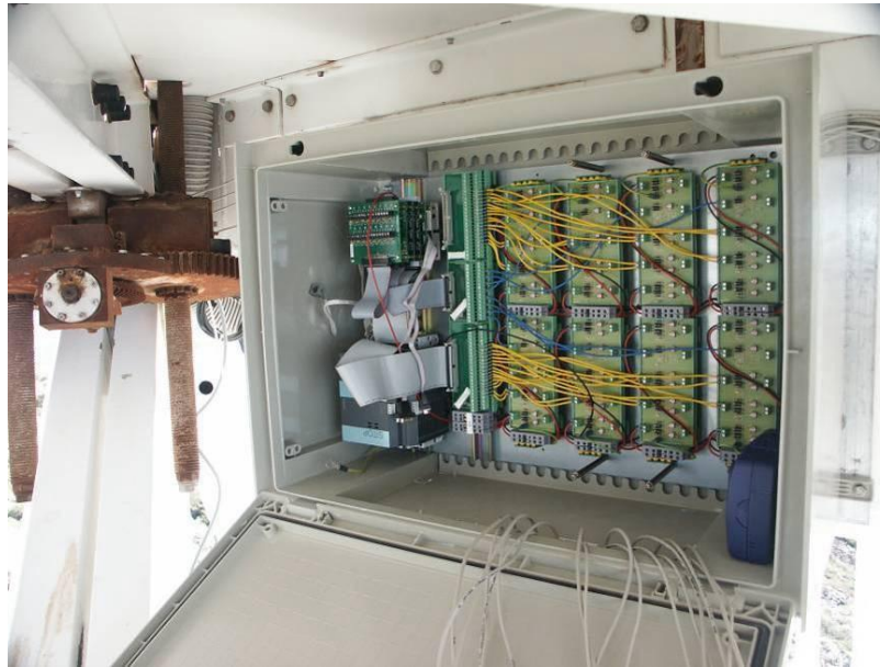
Fig. 9. Anemometer (cups) and vane connection box mounted under the platform floor of the open DOT tower. When closed, the inside of the box is protected against the heavy weather situations of storm combined with rain, snow or ice.
