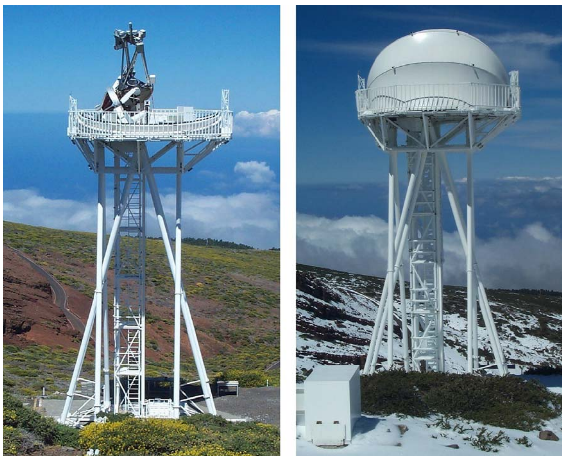
Figure 1. Dutch Open Telescope (DOT) with open-foldable enclosure of cloth segments. Left: enclosure open, leaving the telescope completely free in natural flushing of the wind. Right: enclosure closed with strongly tensioned cloth segments. Practically no snow or ice sticks on the tent cloth due to its smooth coating, whereas much snow and ice are visible in the ladder and elevator framework (see also Figure 3).
