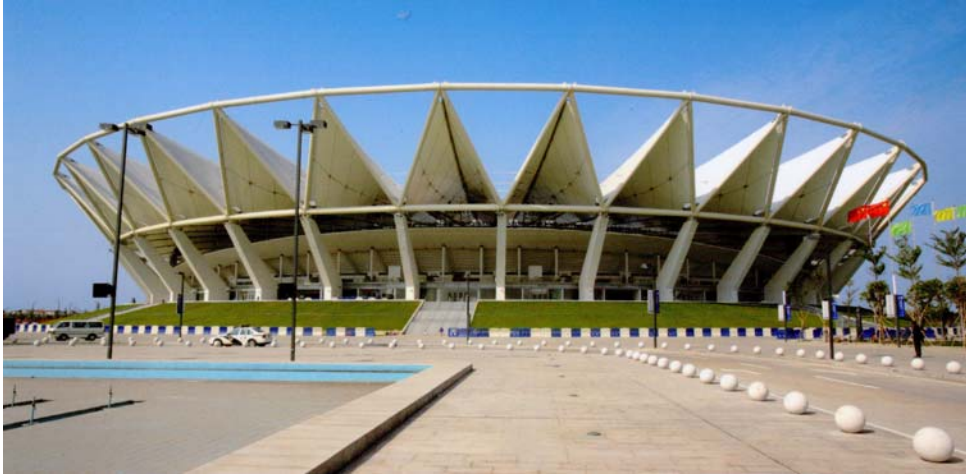
Figure 11. Foshan Olympic Stadium with cloth parts comparable to the size needed for an EST enclosure.
