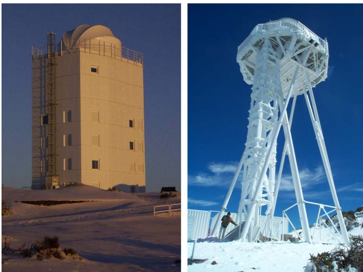
Figure 3. Left: GREGOR after snowfall. On top of the 20-m high tower is the closed, completely open-foldable telescope enclosure of 9-m diameter. On the tent cloth no snow is present because it slides downward over the smooth coating of the cloth. Right: DOT at the same time as shown in the right part of Figure 1, but seen from another side. Snow and ice in ladder and elevator framework are clearly visible from this side. No snow or ice is present on the cloth of the enclosure on top. In addition, the coarse framework of the large tubes remained clean, as the photo shows.
