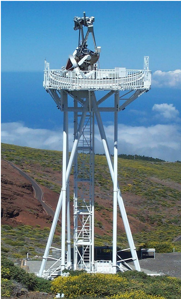
Fig. 4 Dutch Open Telescope (DOT) with open-folded dome of textile membranes between steel bows moved down, leaving the telescope completely free in natural flushing of the wind.
