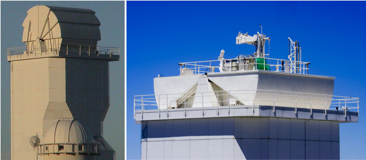
Fig. 1 Vacuum Tower Telescope (VTT) enclosure of open-foldable solid segments. Left : closed with 3 segments visible at each side. Right : open with all segments under the telescope platform.
