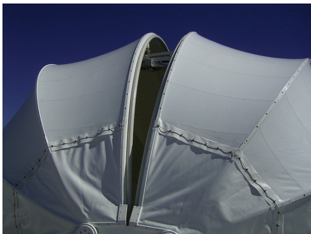
Fig. 12 Start of the opening of the GREGOR dome on top of the building. View to one of the two head ends with drives. Additional membrane parts are put around these regions where the main membranes end. A closed connection is realized between main membranes and the head ends. The upper main membrane parts are still tensioned because of the weight of the in-between bows. This fact contributes to a safe opening and closing during strong wind because it prevents flapping of the upper membranes, which are more exposed to the wind.
