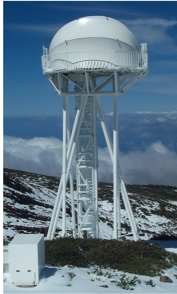
Fig. 5 DOT enclosure in closed position with strongly tensioned cloth segments. Practically no snow or ice sticks on the membranes due to its smooth coating.
