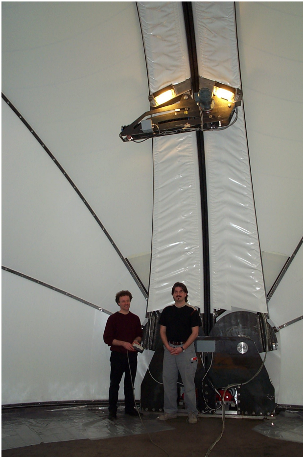
Fig. 9 The closed GREGOR dome seen from the inside during the tests in the workshop DEMO at Delft. The picture shows at the bottom one of the two drive units for the main center bows and on top one of the two clamps, which bring the textile membranes to high tension when the clamps move the two center bows together into their final position in a completely closed dome. The main center bows are covered at the inside by an additional cloth for thermal insulation.
