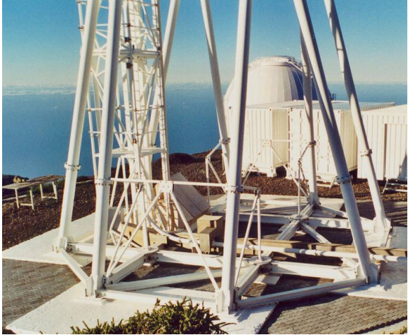
Figure 6: The base of the DOT tower with small perpendicular tubes.
