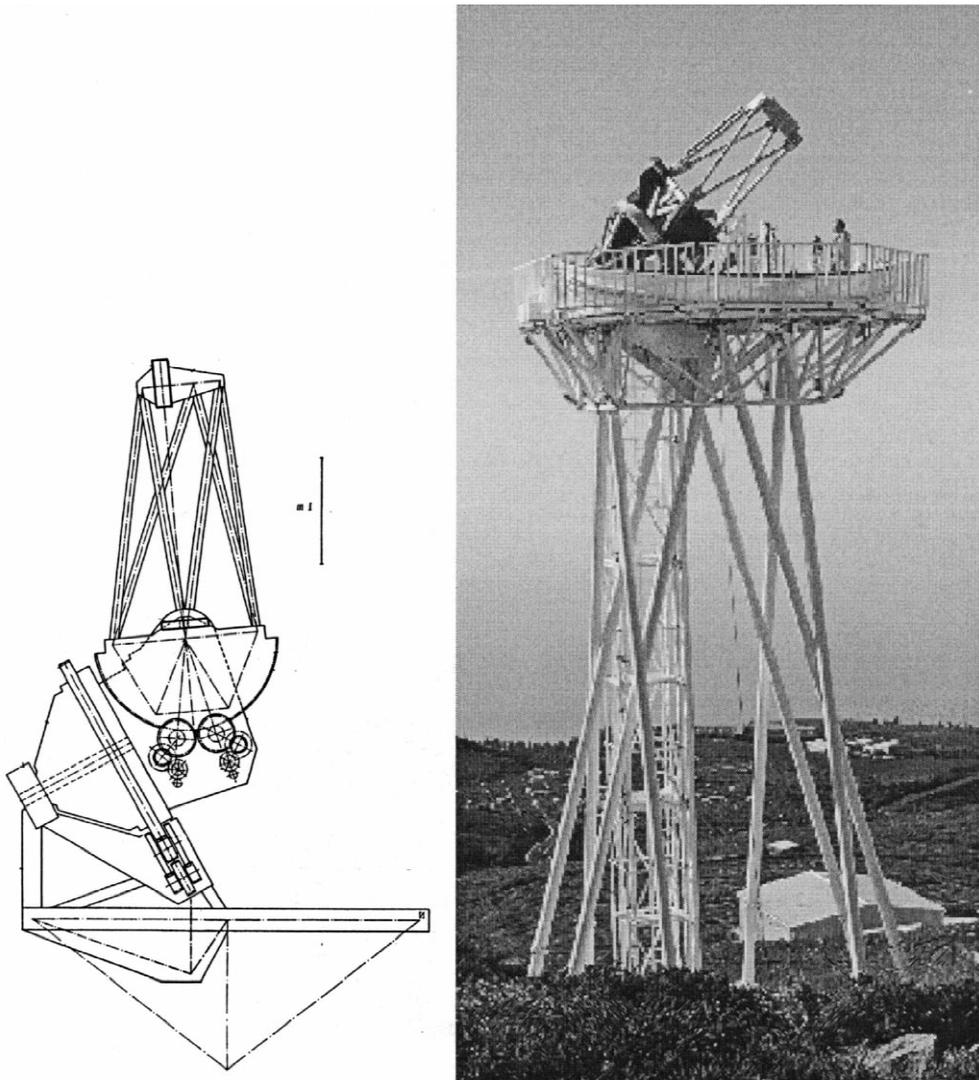
Fig. 1. Left: sketch of the DOT pointing at the Sun at noon on June 21 (La Palma). The bar measures 1 m. Right: the DOT on its tower, 1996 October (La Palma). North is to the right.
