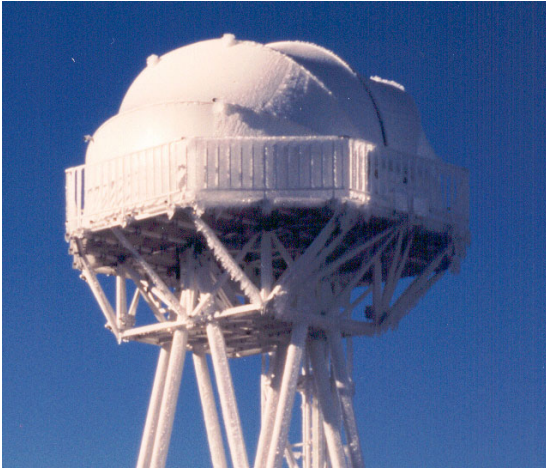
Figure 12: The DOT after ice formation by clouds. The cloth is relatively clean from ice.
